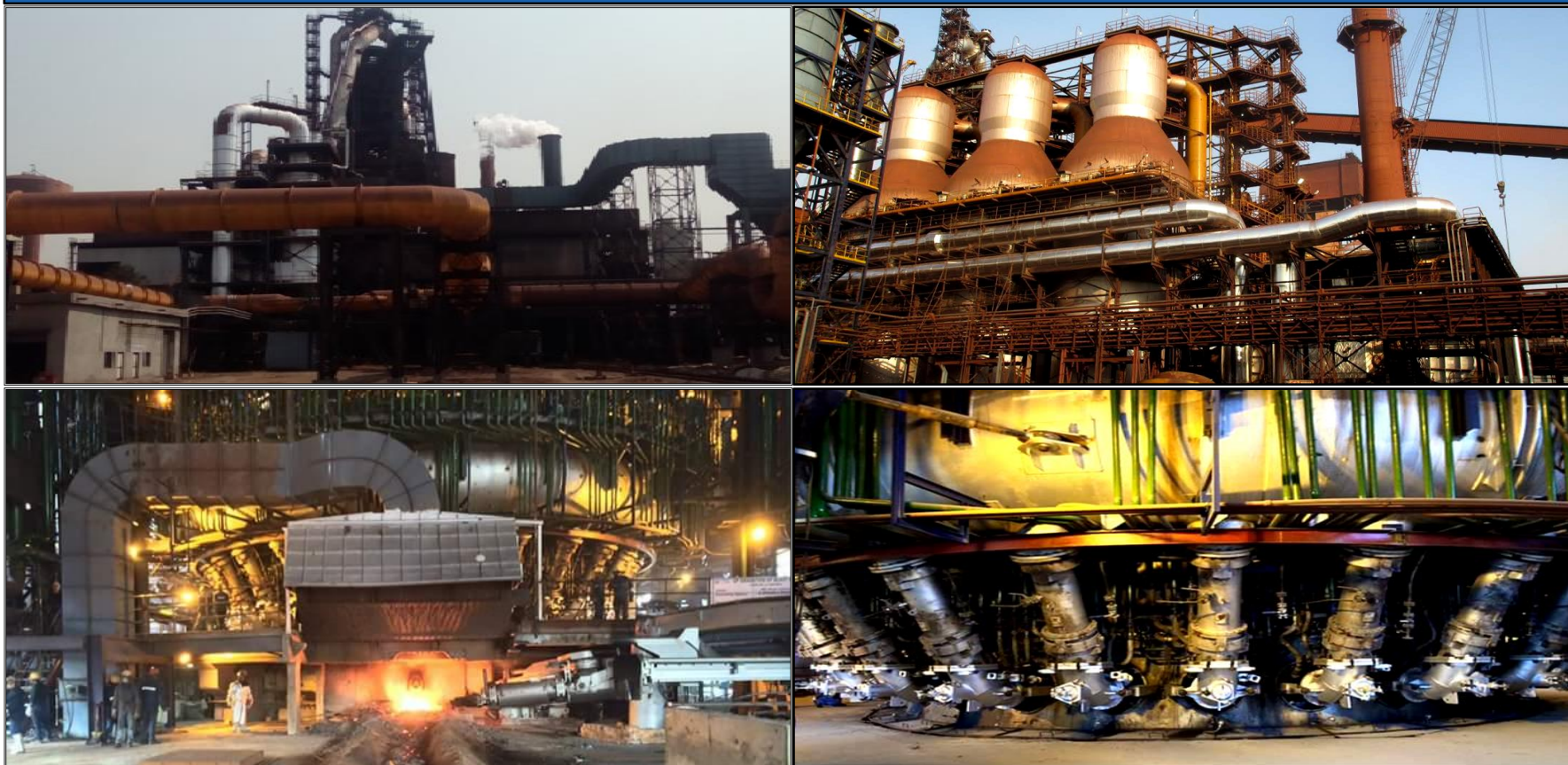
Blast Furnace -1 reconstruction at Vijayanagar: re-commissioned in 4QFY16
